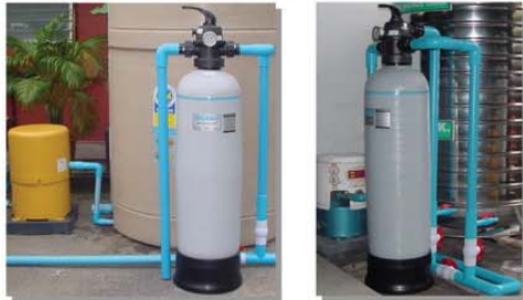
Installations of W300 filters with pressure pumps and water reserved tanks
